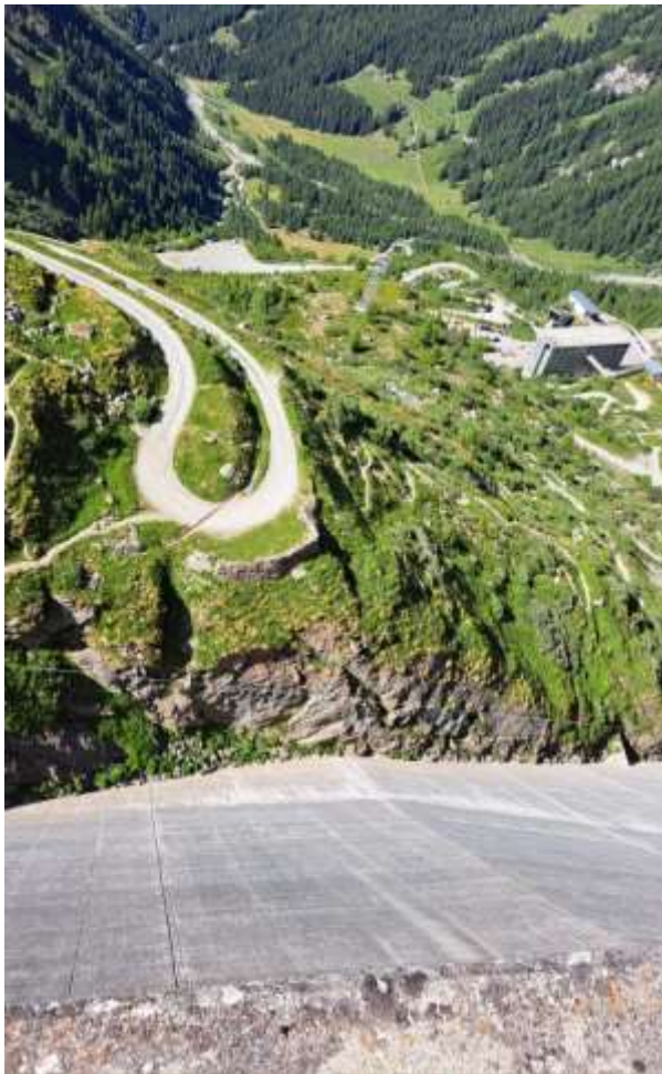
Peering over the side of the dam wall.
